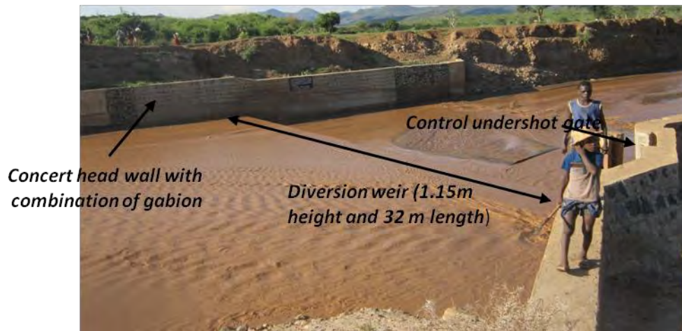
Figure 4-3 Potota diversion structure (Gizachow T., 2013)
