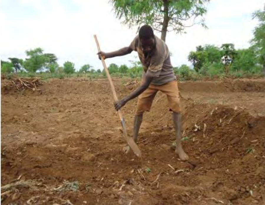
Figure 4-16 Soil bund maintenance at Oneya scheme of Yandafero spate irrigation, 2013
