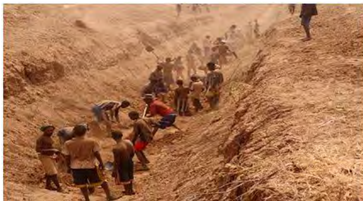
Figure 4-15 Removal of the sediment from the primary canal at Tarakoma scheme, 2013
