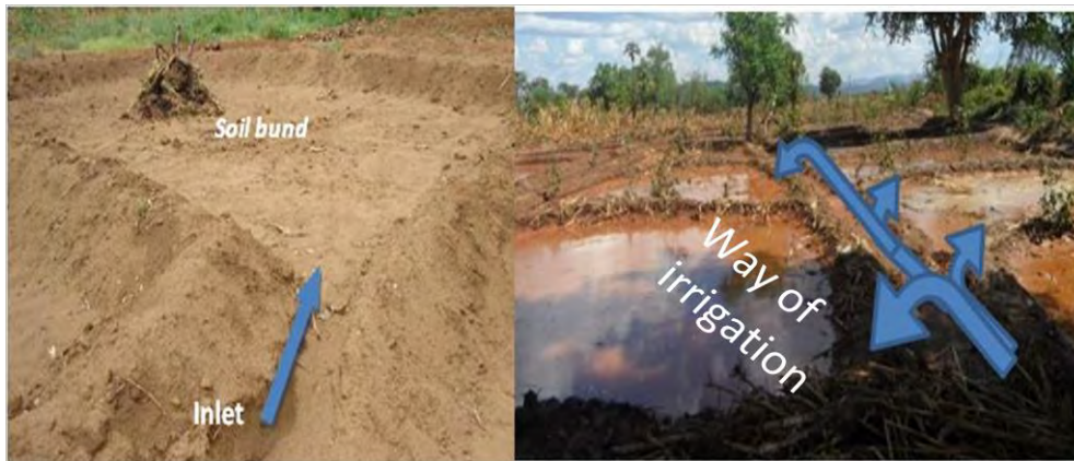
Figure 4-9 Prepared Field bunds at Tarakoma scheme and irrigated fields
