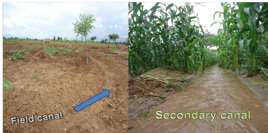
Figure 4-8 Field canal and flood water flow through secondary in Oneya scheme
