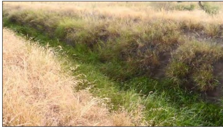
Figure 4-21: Closed of the primary canal in Potota scheme by grass and sediments, 2013
