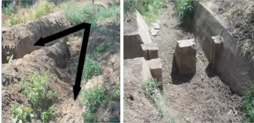
Figure 4-7 Traditional (left) and improved (right) flood flow division structure at Oneya scheme, 2013
